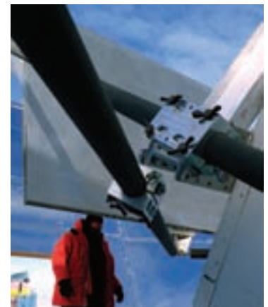
GMT support structure for the Keck Array.
